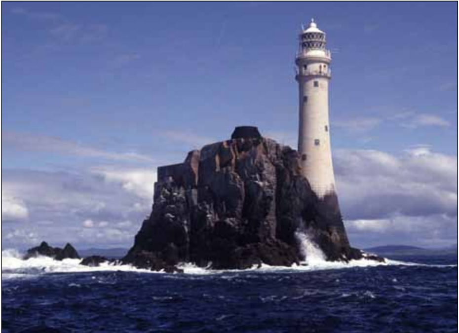
The Fastnet Rock and its lighthouse, (photo: Dick Coombes).
